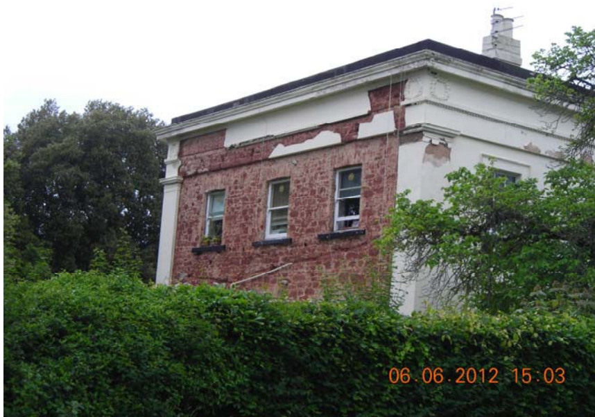
South east elevation showing removal of render
